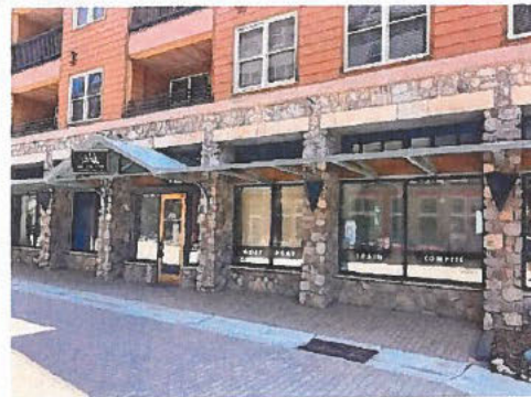
EXTERIOR ENTRY VIEW
