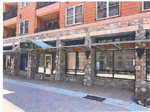
EXTERIOR ENTRY VIEW
